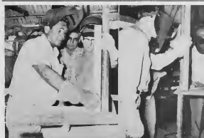
PRECISION WELDING is checked with a square by Gabriel Ruiz. Instructor Morris checks the job, while M. S. Bistlick watches the procedures (left). At right, Modesto Figueroa gets the feeling of the welding rod. A welding mask is essential for eye protection. The welding class began April 4 for the first group.
